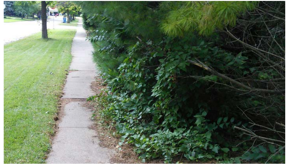
In this block of sidewalk, vegetation overgrowth acts as an obstruction and reduces the passable width to 39 inches. The largest vertical fault on the block is over 1/2 inch, and the maximum cross slope is 10 percent, resulting in a combined compliance score of 15.
