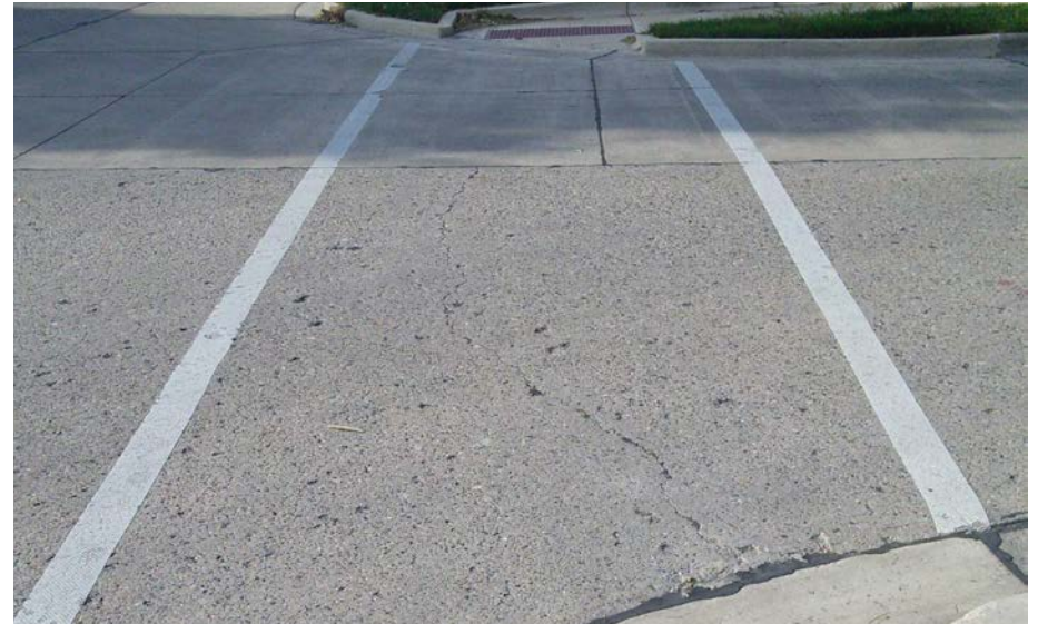
This crosswalk at an uncontrolled intersection scores 100 on the compliance index due to its width of 91 inches and its cross slope of 0.7 percent.
