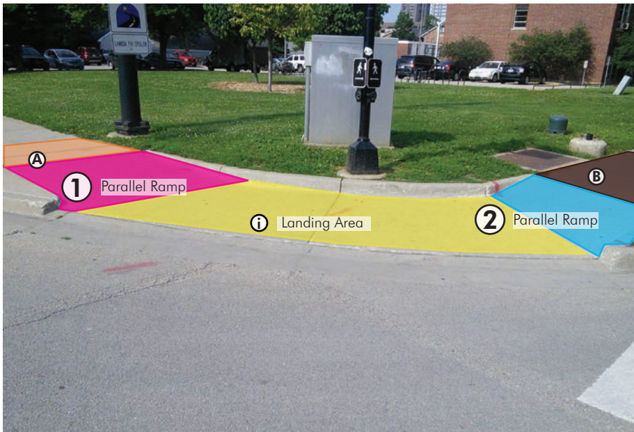
Figure A-7 Approaches for Parallel Ramps
