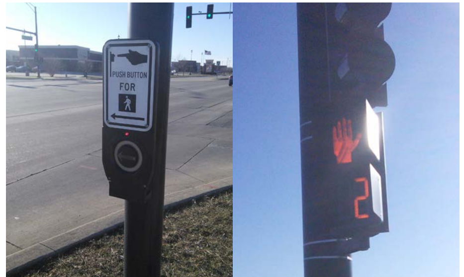
Though the signal itself is similar to the previous example, this pushbutton has all of the required accessibility features and scores 100 on the compliance index.
