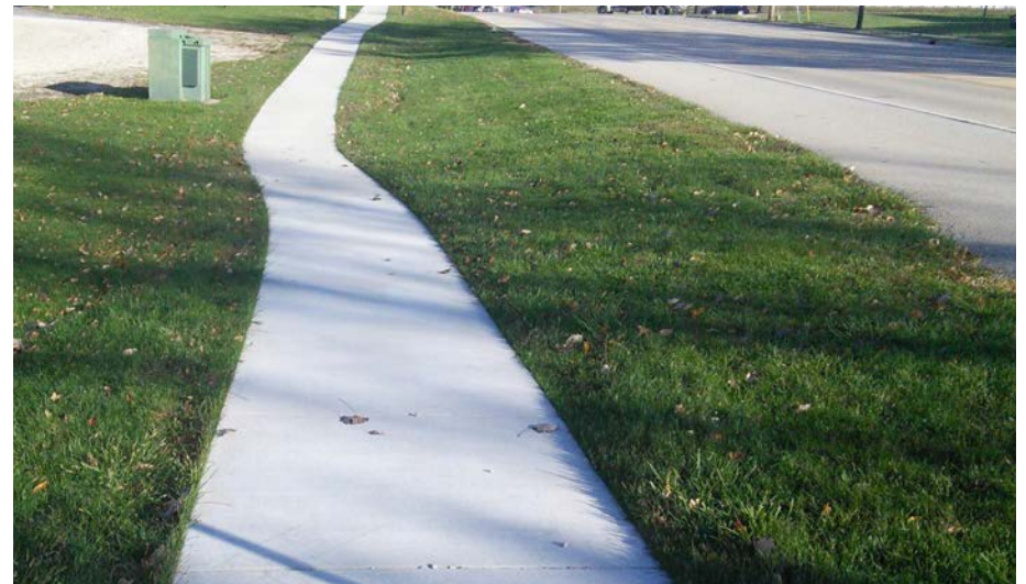
This block of sidewalk is 60 inches wide and has no vertical faults or obstructions. With a maximum cross slope of 2.3 percent, it scores 95 on the combined compliance index.
