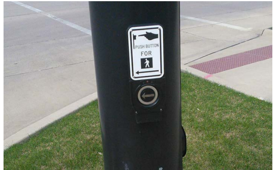
This pushbutton has a variety of accessibility features and appears to be in good condition, but field staff noted that it was not operable.
